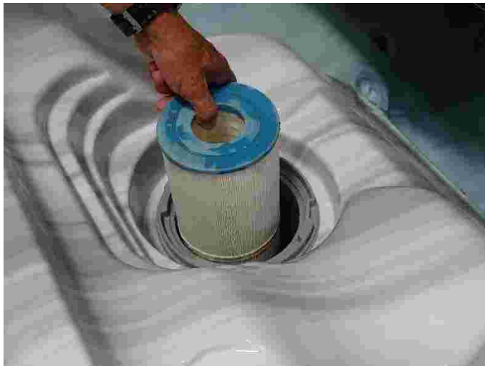
Figure 16. Drop in filter removal
