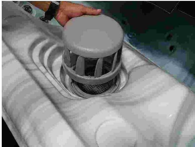
Figure 14. Weir cap removal
