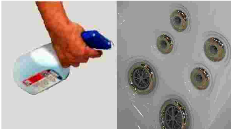
Figure 11. Spraying the jets
