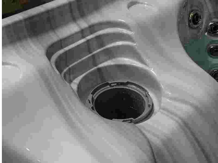
Figure 17. Empty filter housing
